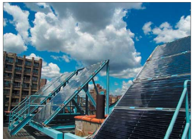
This 64-panel array of Solargenix CPC Collectors serves a mixed-use building in New York City. Photo: Solargenix Energy, LLC
