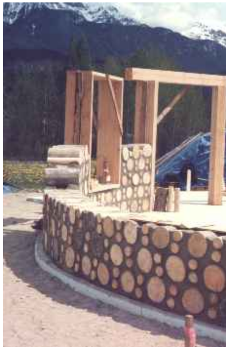
Figure 22. B.C. Cordwood Walls under Construction Source: Earthwood Building School
