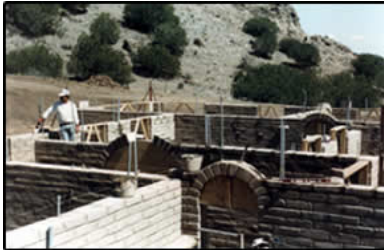
Figure 17. Texas Adobe Under Construction Source: Adobe Builder.com
