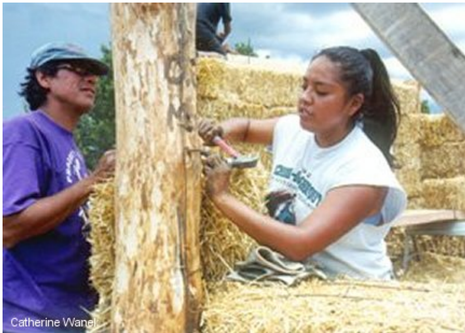
Figure 19. New Mexico Aboriginal Workshop in Infill Strawbale Source: Strawbale Group / Builders Without Borders
